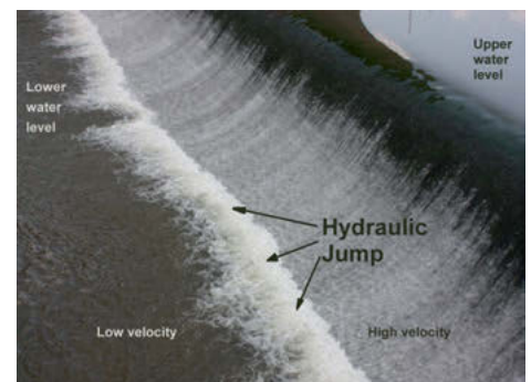
Hydraulic jump at spillway
