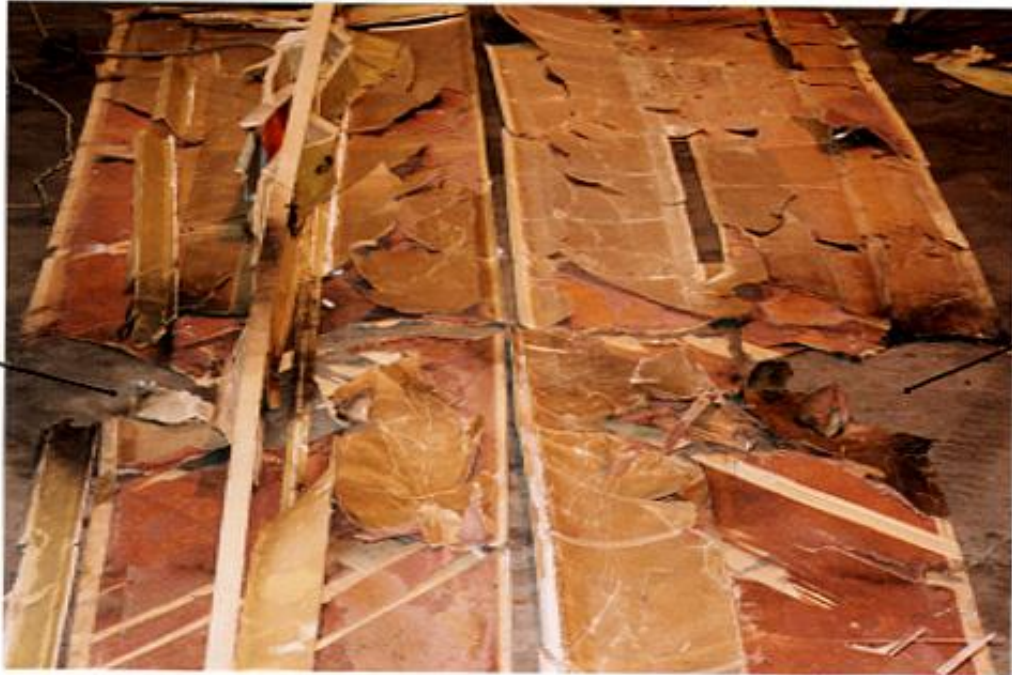
Detail of right wing structure in region of aileron actuator rod/bellcrank*
