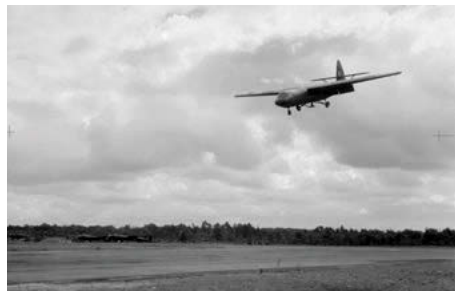
A Horsa Mark I coming in to land, with "barn door" flaps down, at Portreath, Cornwall, in 1943
