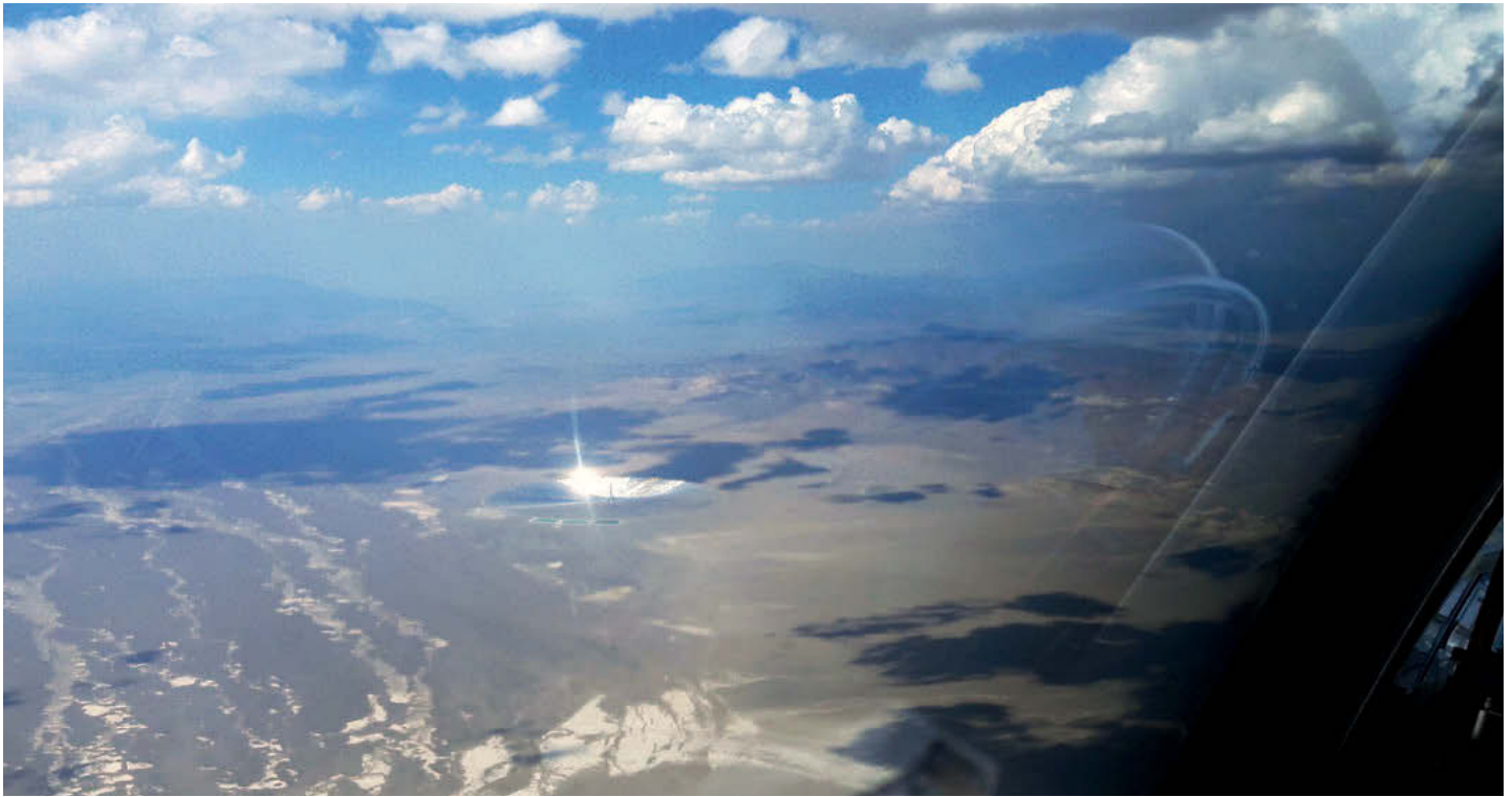
Crescent Dunes solar power station – over 10,000 large mirrors set in a 1,600-acre circle with a 700ft tower in the centre
